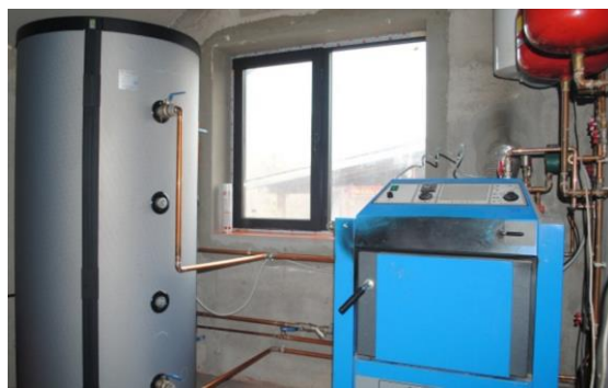
Figura 12. Boilerul mixt instalat in camera centralei termice
