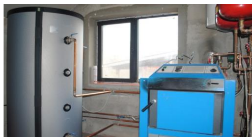
Figura 12. Boilerul mixt instalat in camera centralei termice
